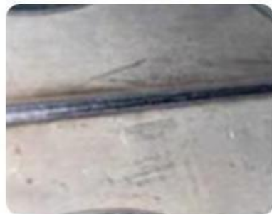
CARBON STEEL FLAT WELDING
